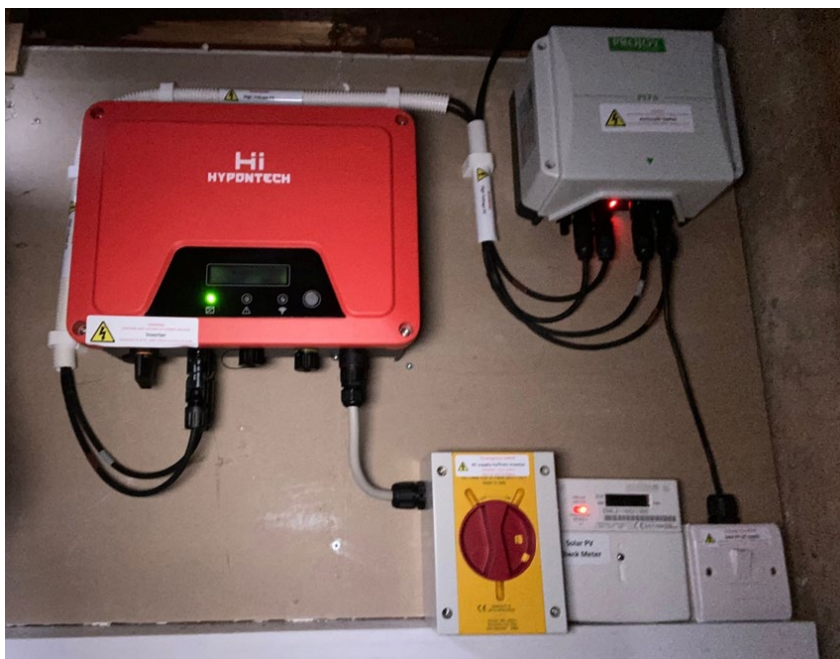
Figure 13. Solar inverter and electricity meter
