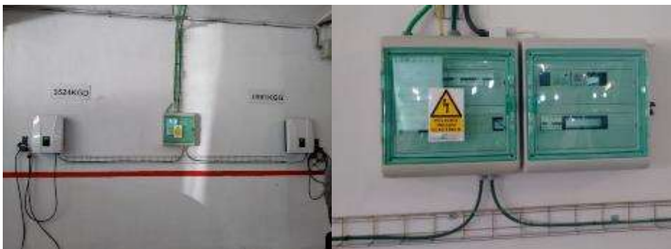
Figure 4. Installation of meters and controllers for the electric cars' charging point.
