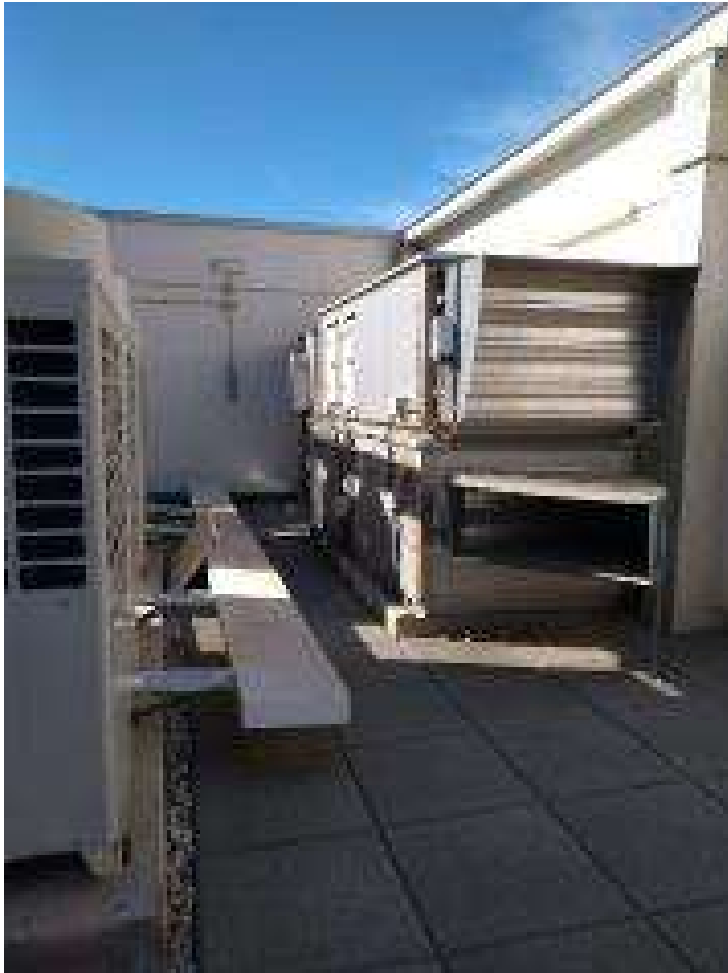
Figure 5. Photograph of the room of the building with the compressors of the conditioning system on the left and the Air Handling Unit in the right.
